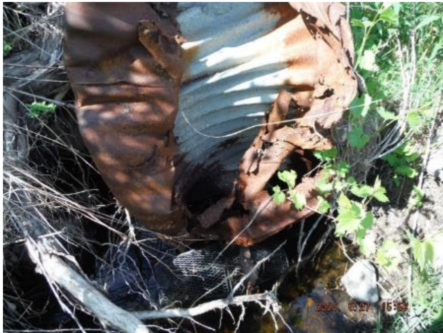
Photo 27: Culvert at access road (May 27, 2020)
