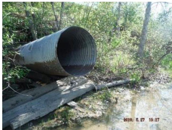
Photo 35: Culvert Under Railroad at Headwater Feature 2 (May 27, 2020)
