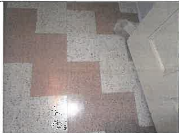
Photo 11: 8" floor tile (Type C– White and reddish tile with spots) observed in Room 19 (Asbestos).
