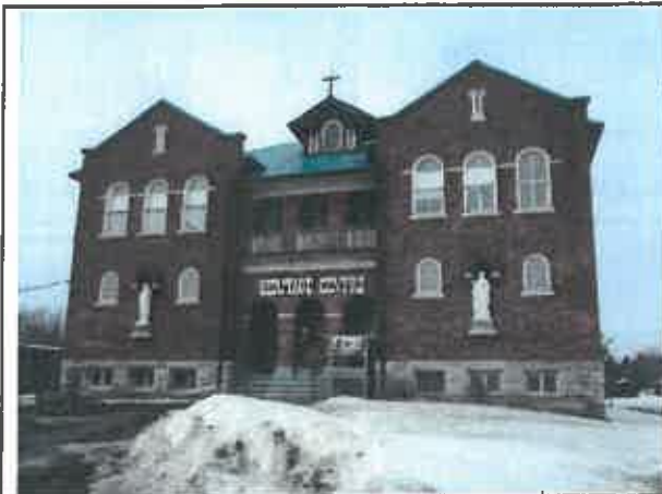
Photo 1: St Andrews Library and Museum building exterior.
