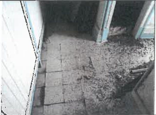
Photo 17: 8" floor tile (Type F— pink and green streaks) observed in Room 27 (Non-Asbestos).
