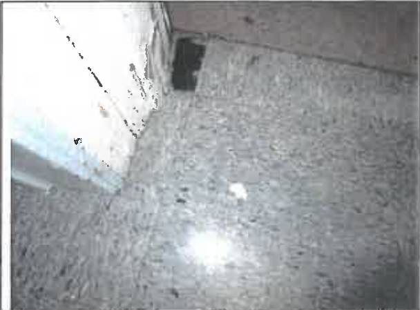
Photo 20: 12" floor tile (Type B – grey and white fleck) observed in Room 4 (Non-Asbestos)
