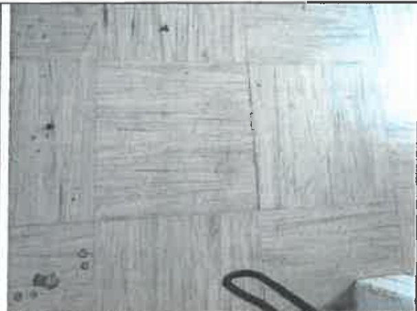
Photo 14: 8" floor tile (Type E— pink and green) observed in Room 20 (Non-Asbestos).
