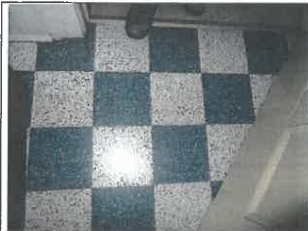
Photo 7: 8" floor tile (Type A – Green and White) observed in Room 10 (Non-Asbestos).
