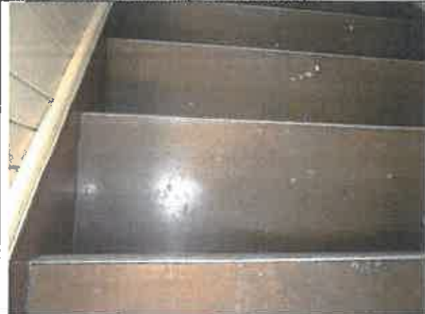
Photo 9: Linoleum (Type A – Brown) observed in Room 15 (Non-Asbestos).
