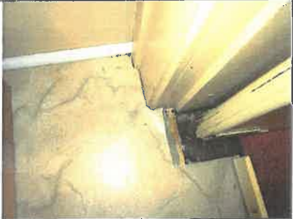
Photo 4: linoleum (Type A – beige marble pattern) observed in Room 2 (Non-Asbestos).
