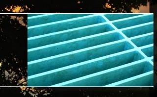
Bar intake pipe and clogging it. The special coating helps to prevent gate valve. the formation of any frazil ice that could potentially clog or jam the bar screen.
