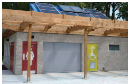
Public Washroom Building
