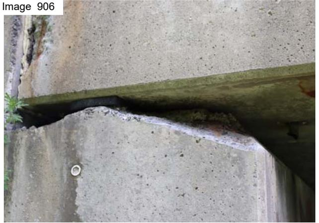
NW bearing seat disintegration
