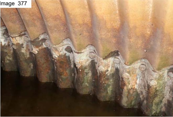
Waterline corrosion at west
