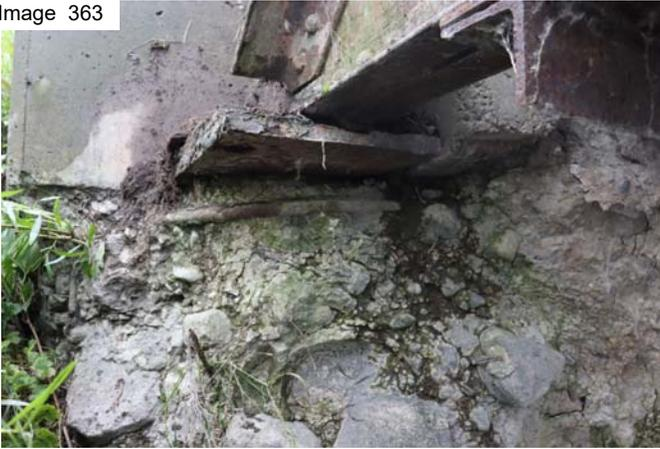
SE bearing abutment disintegration
