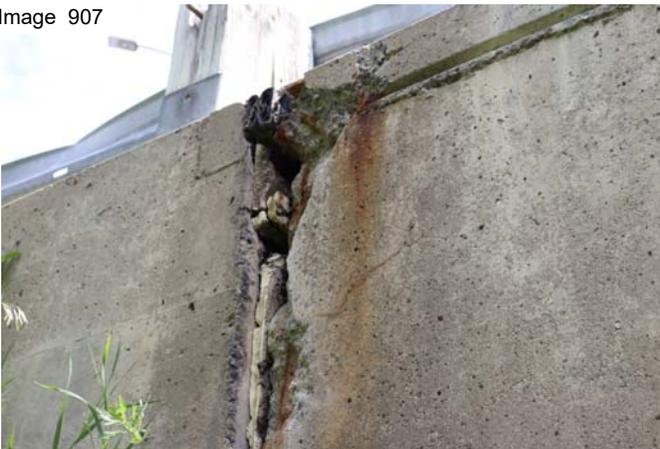
NW corner disintegration under expansion joint
