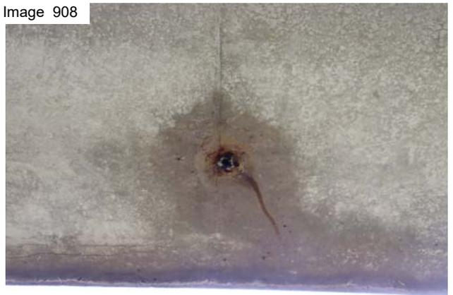
Deck drain end with saturation and rust (typical)
