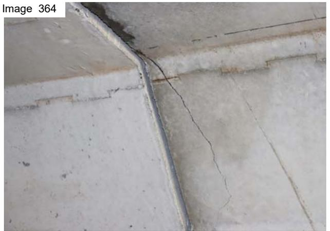
Crack in west wall
