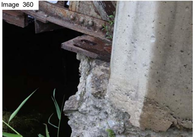
SW bearing disintegrating abutment
