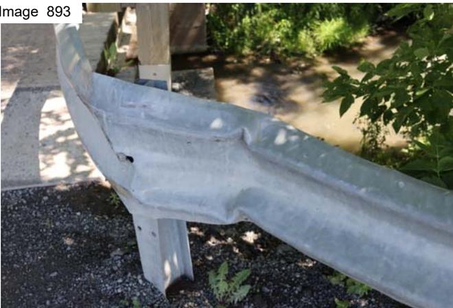
Guide rail damage SE
