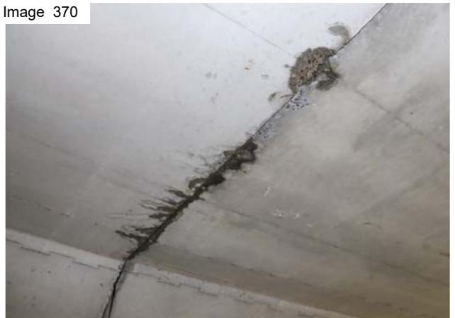
Leaking at joints
