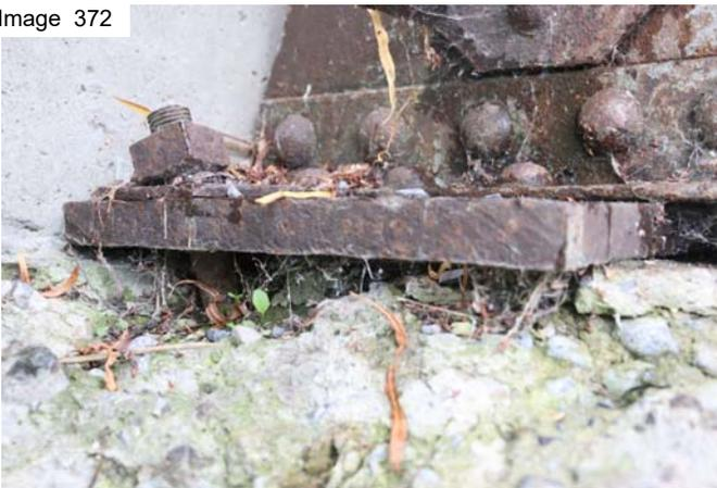
NW bearing missing bolt
