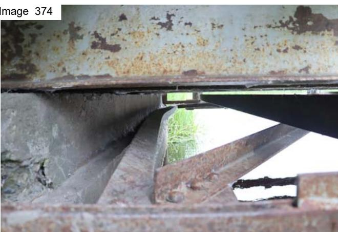
Bent lateral brace north abutment
