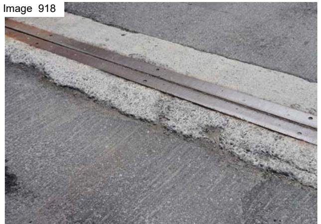
North expansion joint end dam damage
