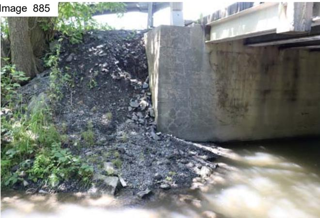
Erosion in SE embankment
