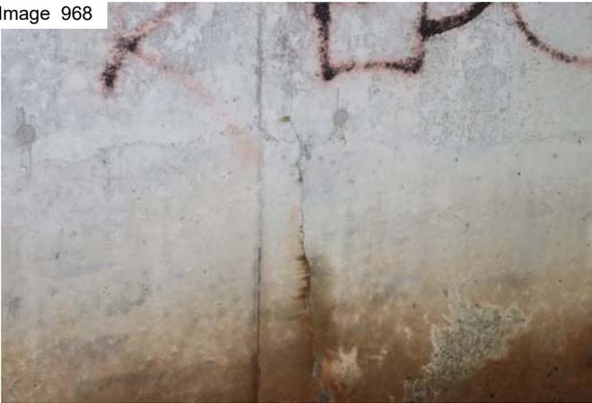
Horizontal and vertical cracking in west abutment
