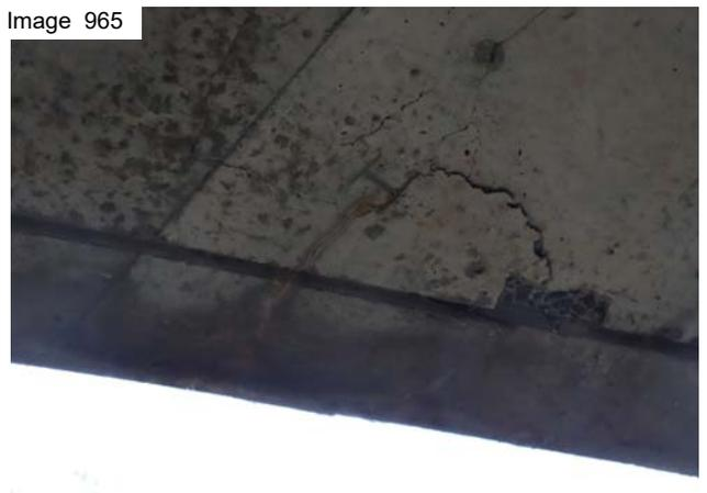
Delamination in south soffit
