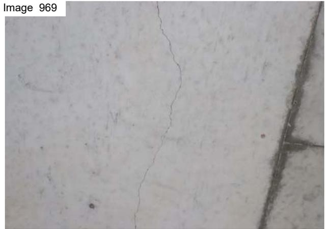
Small soffit crack
