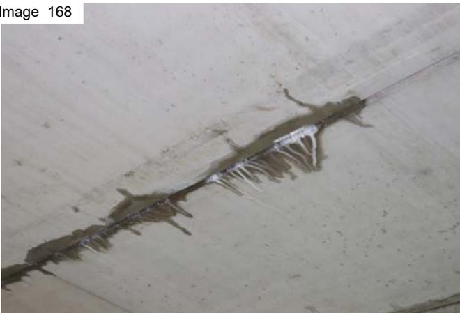
Soffit joint leaching and saturation
