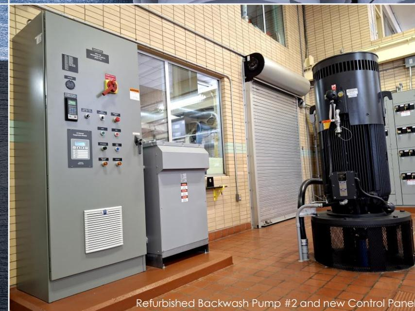
Refurbished Backwash Pump #2 and new Control Panel.
